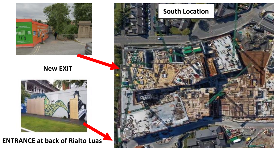
Figure 1 South Side Location at Rialto Bridge and Luas Stop
