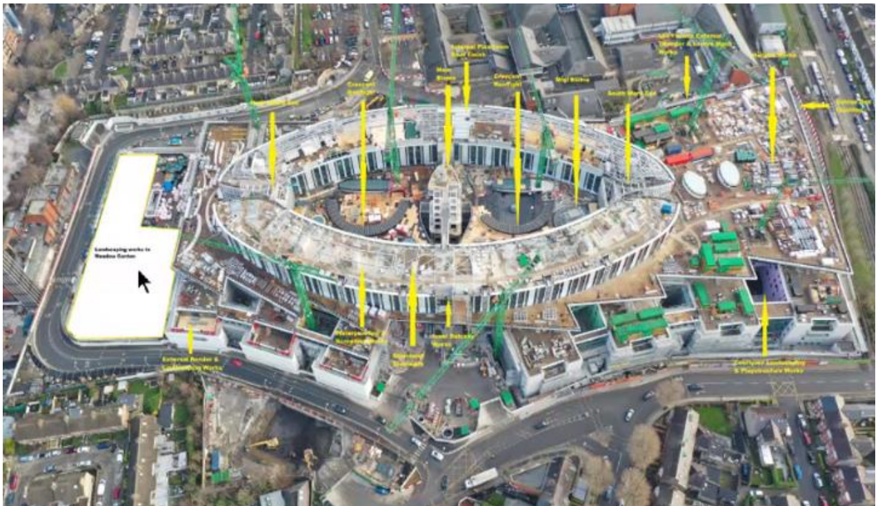
Figure 1 Drone shot of structure from SCR March2
